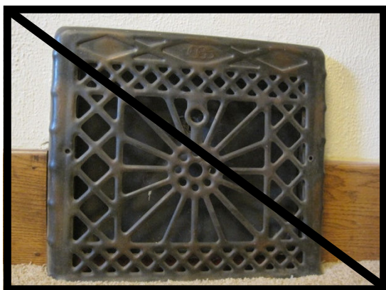
1. Hot air registers—dry, heated air blowing directly on the back of a piano is particularly bad for the soundboard.
